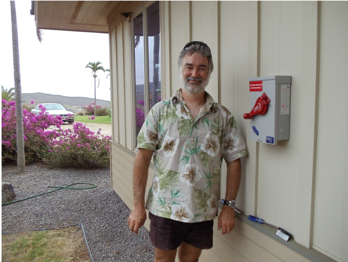
Figure 7 Our happy installer, Tom Carpenter.
