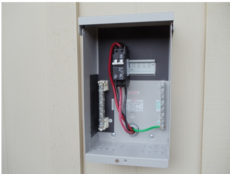
Figure 4 The Midnite MNPV6 Disco enclosure installed in place of the pull switch. A 2 pole 30 amp AC breaker is installed in the enclosure (MNEAC30-2P). The Neutral busbar is not used in this installation.
