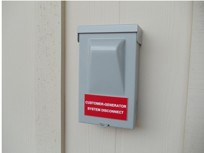
Figure 1 Square D pull switch. Works fine, just not what the customer wanted.
