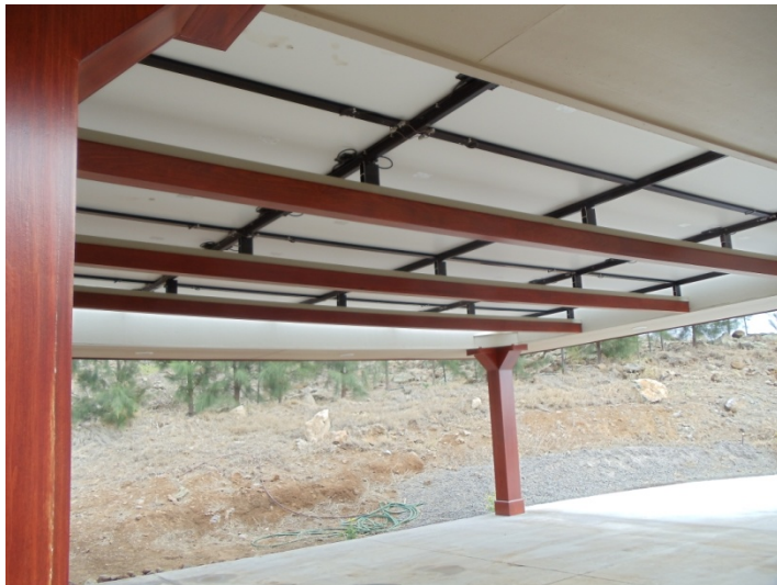
Figure 8 Underside of the 5000 watt array. The customer wished for a carport style array where the solar panels do not show. This reduces output and requires additional module cleaning.
