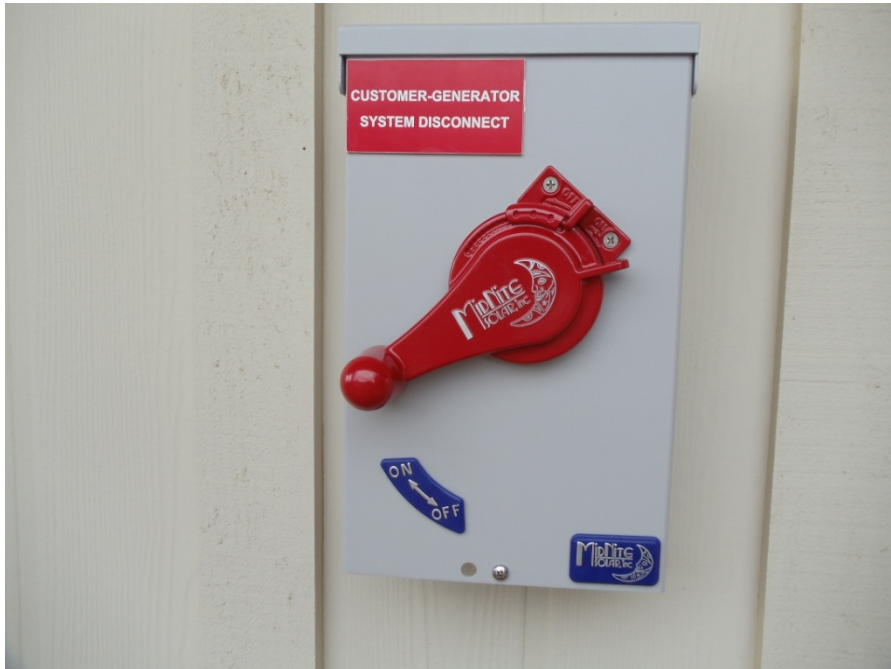
Figure 6 The cover/handle assembly installed with disconnect plaque reinstalled onto the new MidNite disconnect.
